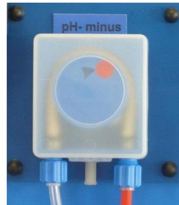
Figure 12, Acid dosing pump
